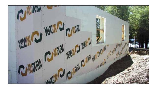
During cold weather months the adhesive formula is modified to allow for lower temperature workability. A protection layer is recommended if coarse material is used for backfilling.
