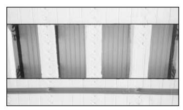
Fasten starter strip on the bottom line with drywall screws at 16" (406mm) c/c.
