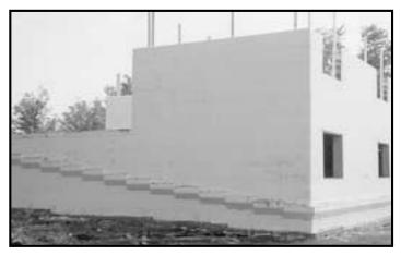
Step of any height increments in the BLE can accommodate any brick or stone size. This feature can prove to be very useful for supporting entry slabs and other applications. It should be noted that different elevations will require different stirrups.
