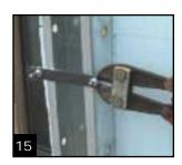
Attach diagonal brace to adapter inserting bolt and nut assembly. Install catwalk and safety guard rails as specified. (fig. 14 & 15)
