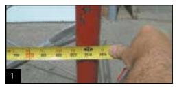
Before starting the first course of forms the installer needs to measure the width of the frame scaffold being used for the tall wall adapter kit. (fig.1)
