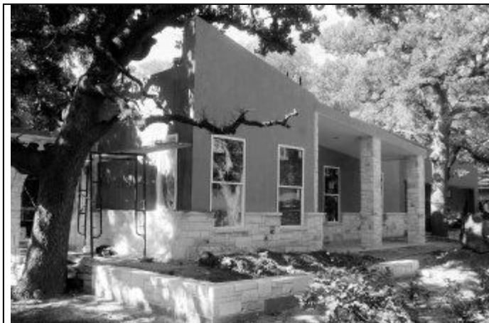
Larry Smith's 4,000-square-foot north Arlington home was built with insulated concrete form, or ICF, construction.
